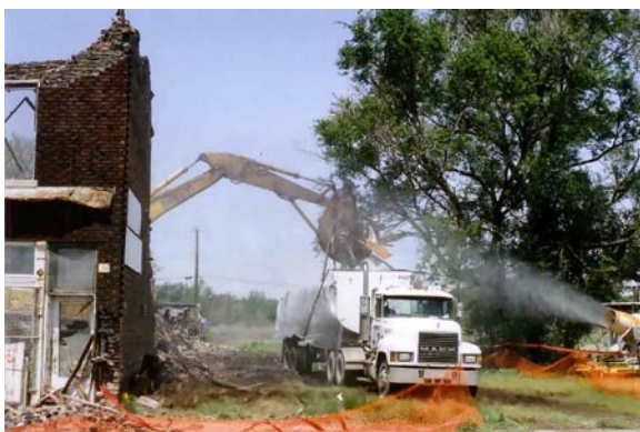
Demolition underway at the hardware store in East St. Louis
